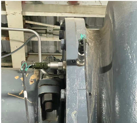
X, Y, Z vibration sensors mounted on compressor
